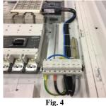
NOTE: - Disconnect the supply to the device or unplug the protective module before performing a resistance test on the system. Otherwise inaccurate measurements are possible. Reconnect the supply /re-insert the module into the base element after the insulation resistance test.
