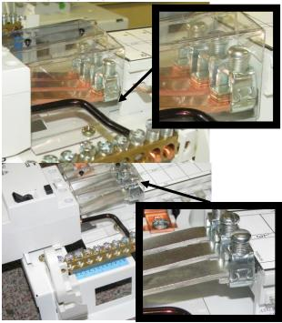
Fit the insulated neutral link to the RCD / Isolator Neutral terminal and tighten to hold. NOTE - For new type baseplate use short link, for old
