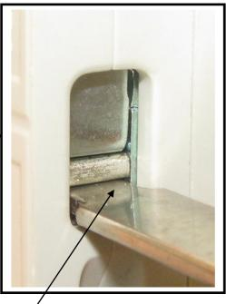
Busbar connection into lower cage, ensure cage is fully lowered before attaching to busbar
