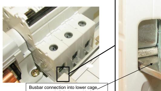
Busbar connection into lower cage, ensure cage is fully lowered before attaching to busbar
