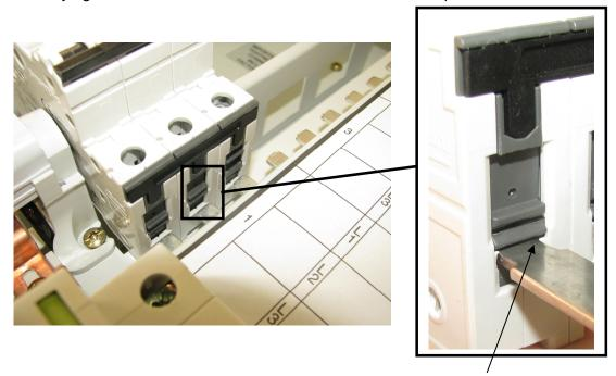
Busbar connection into lower cage, ensure cage is fully lowered before attaching to busbar
